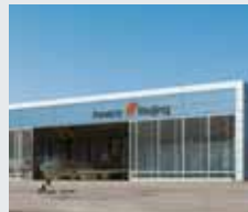
Ameco A380 Hangar Peking, China
